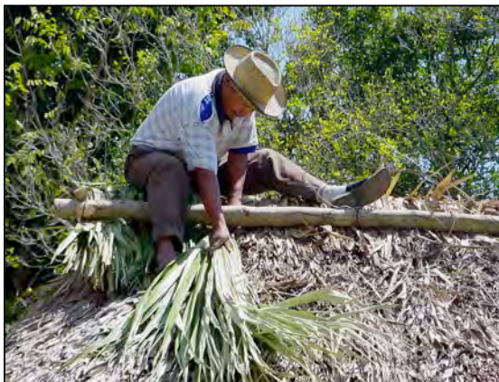
Construction of a palm roof
